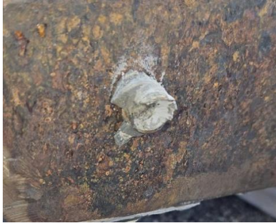
Pic 6: Bolt # 2, Comment: Bolt strongly corroded for some time. Broken and no holding function.
